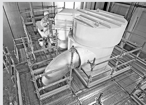
Working scaffolds industry
