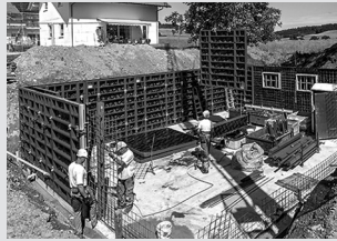
Wall formwork
