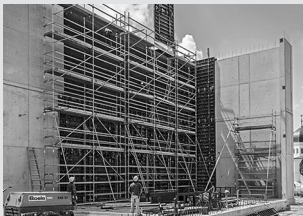
Working scaffolds construction
