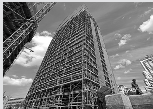
Working scaffolds facade
